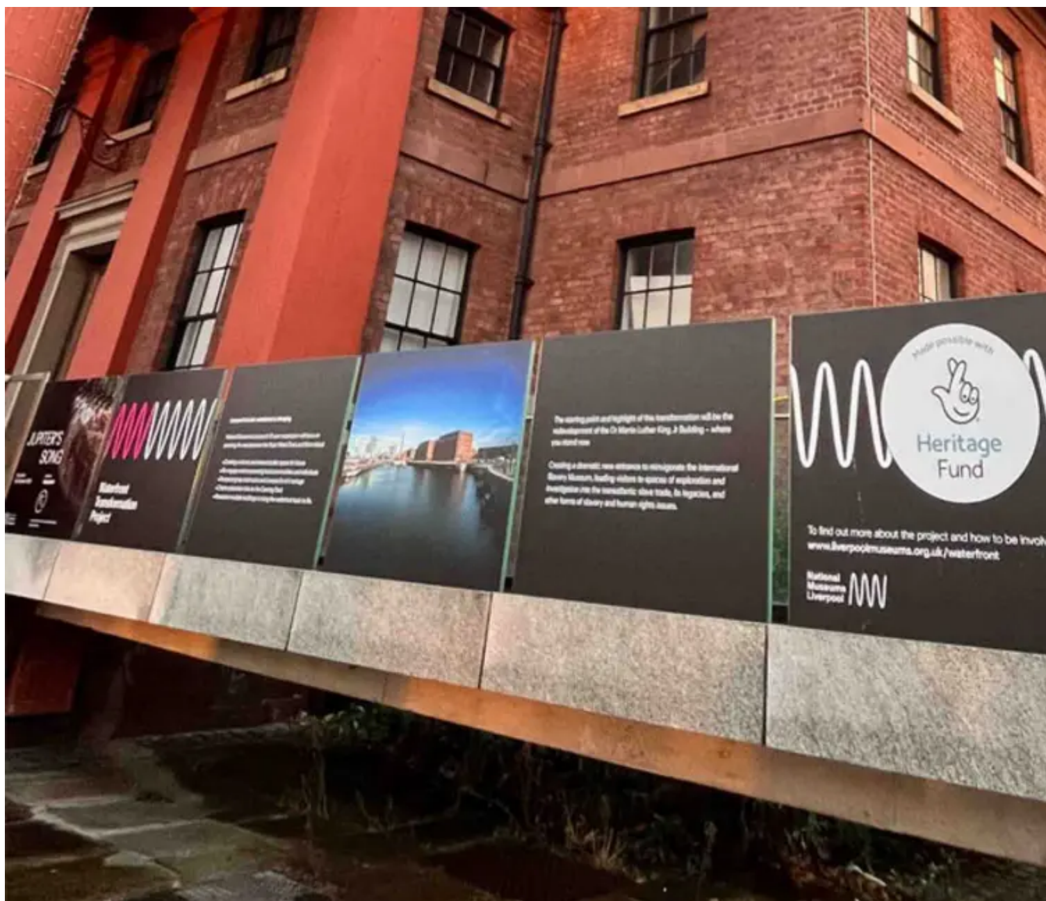
Construction work hoardings.
