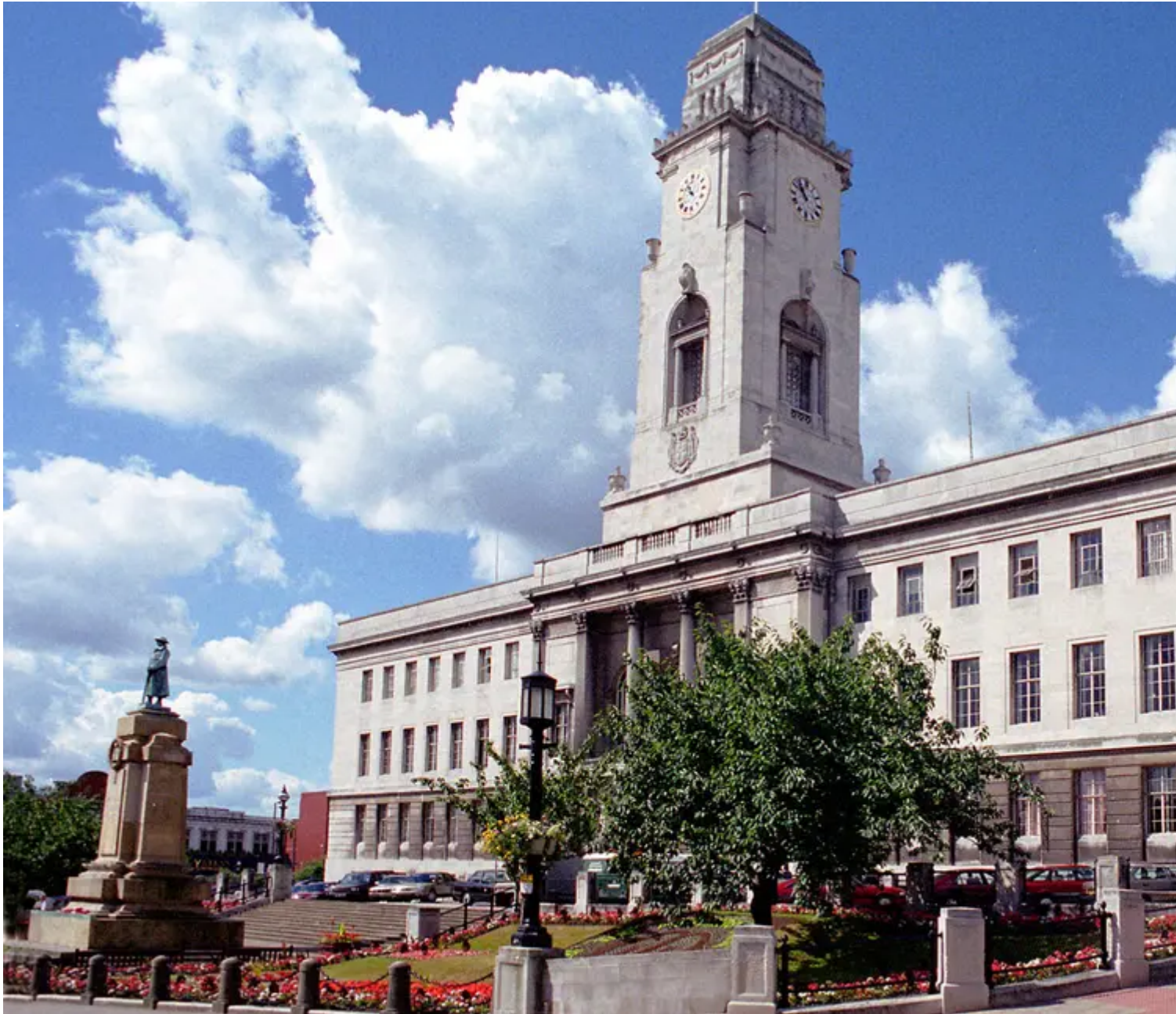
Barnsley's historic Town Hall
