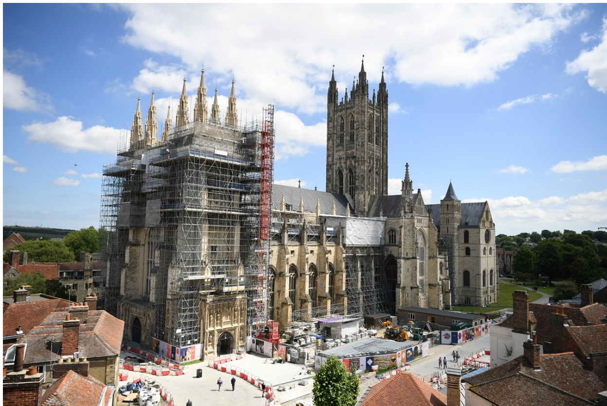
Canterbury Cathedral undergoing restoration
