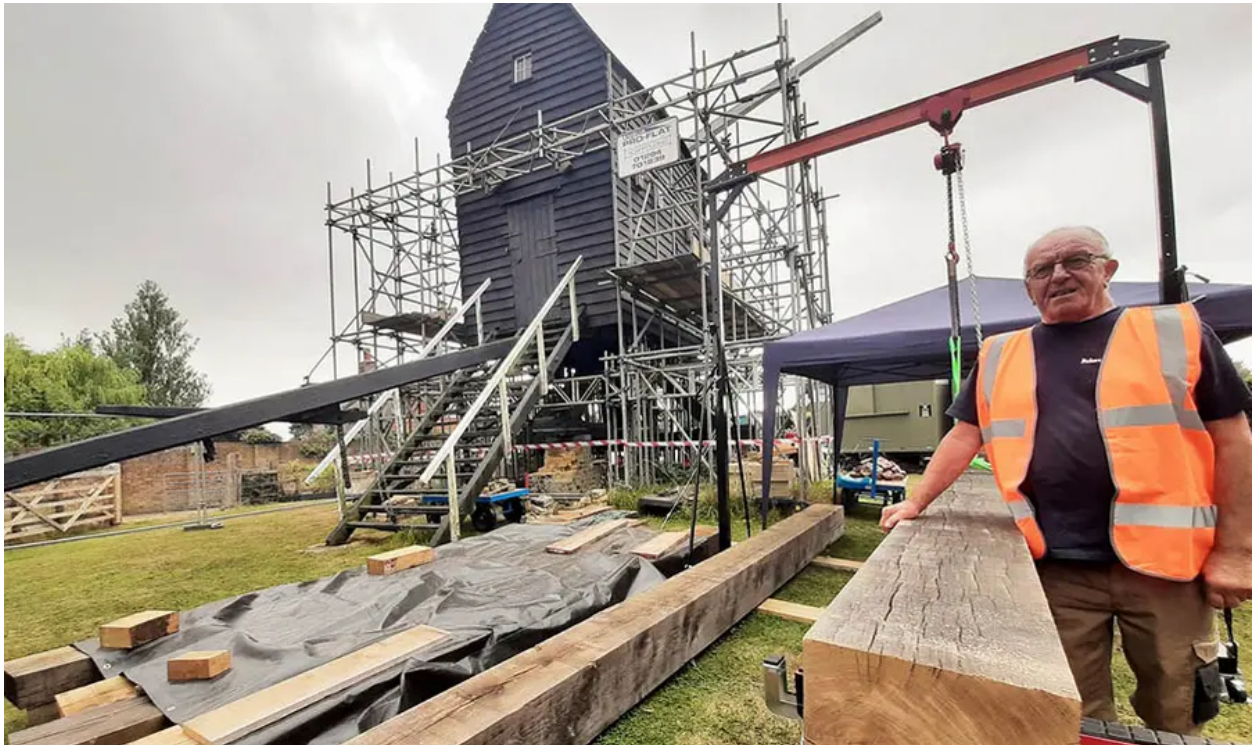
Scaffolding lifted the mill while the huge oak beams that support it were replaced.
